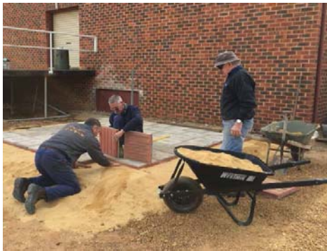
Preparation of shed pad
