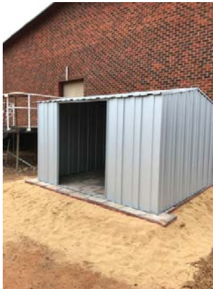
The (almost) finished shed
